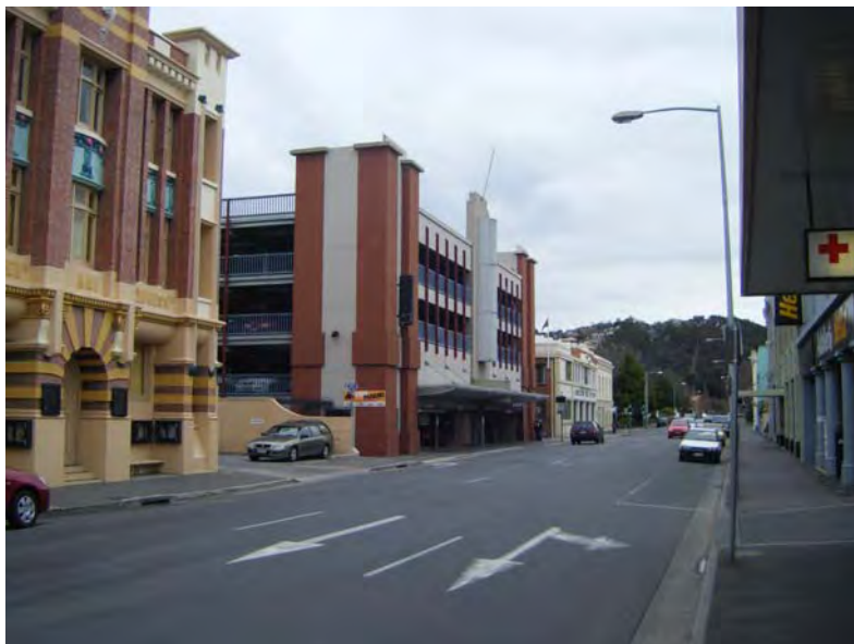
Figure 4: Poor wayfinding to Council's Paterson St. East car park
