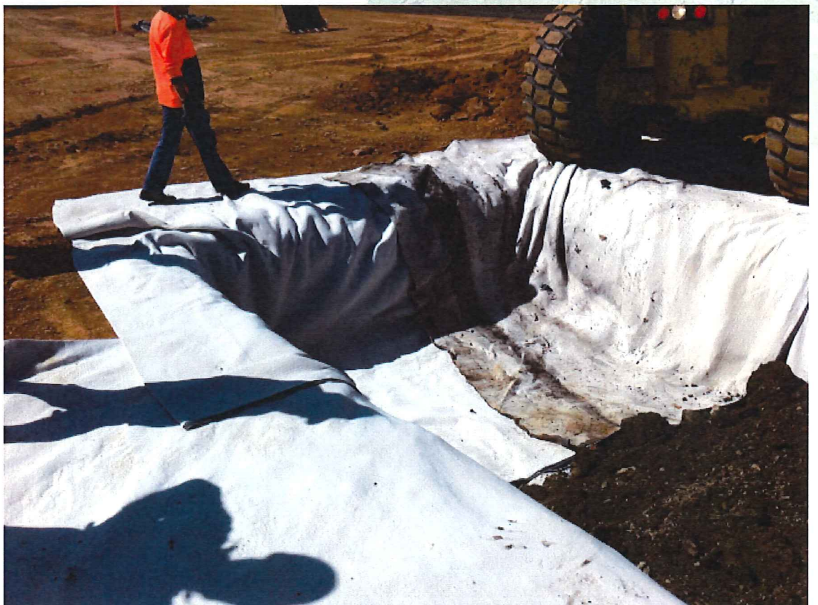
Figure 4: End of Trench, note geotextile fabric overlapping the end of the trench.
