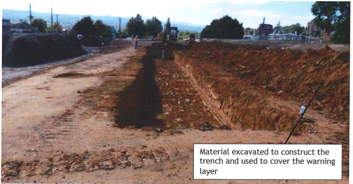
Figure 1: Excavation of the trench
