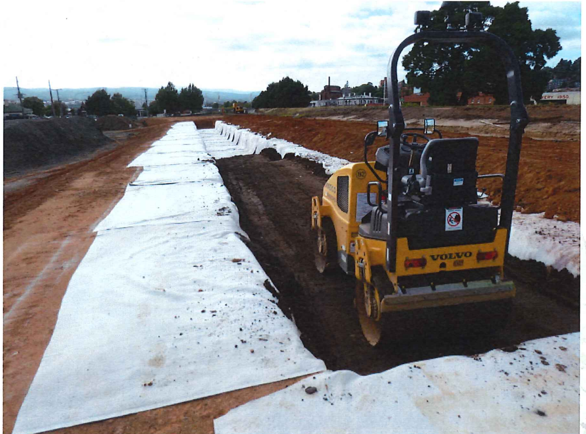
Figure 3: Placement and rolling of material in trench.
