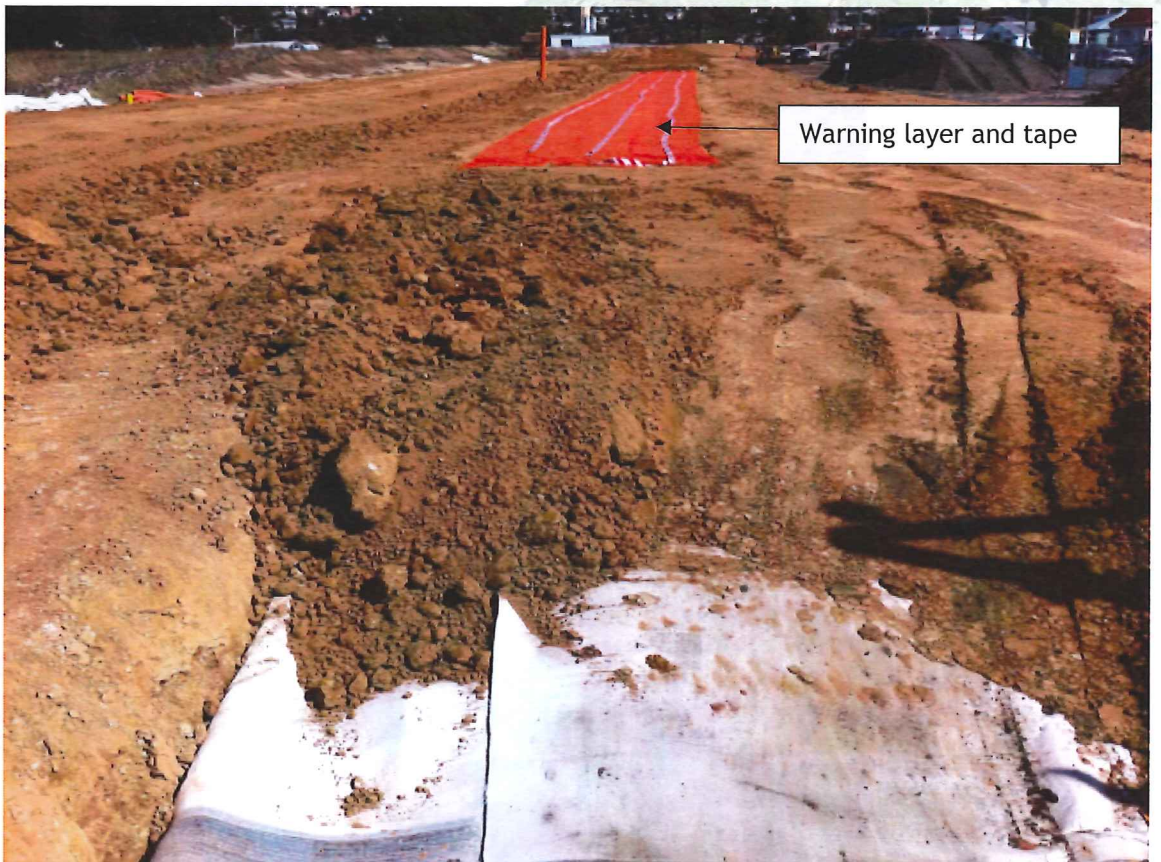
Figure 6: Placement of Clay and warning layer of wrapped material.
