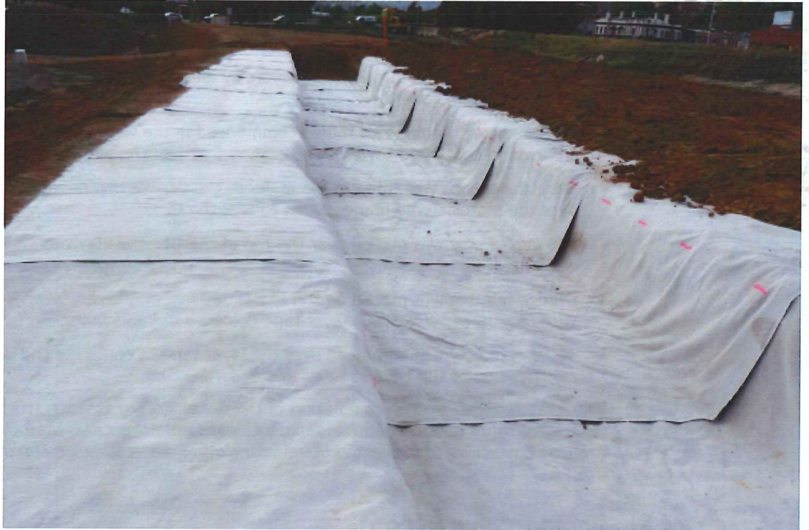
Figure 2: Placement of Geotextile Fabric in Trench
