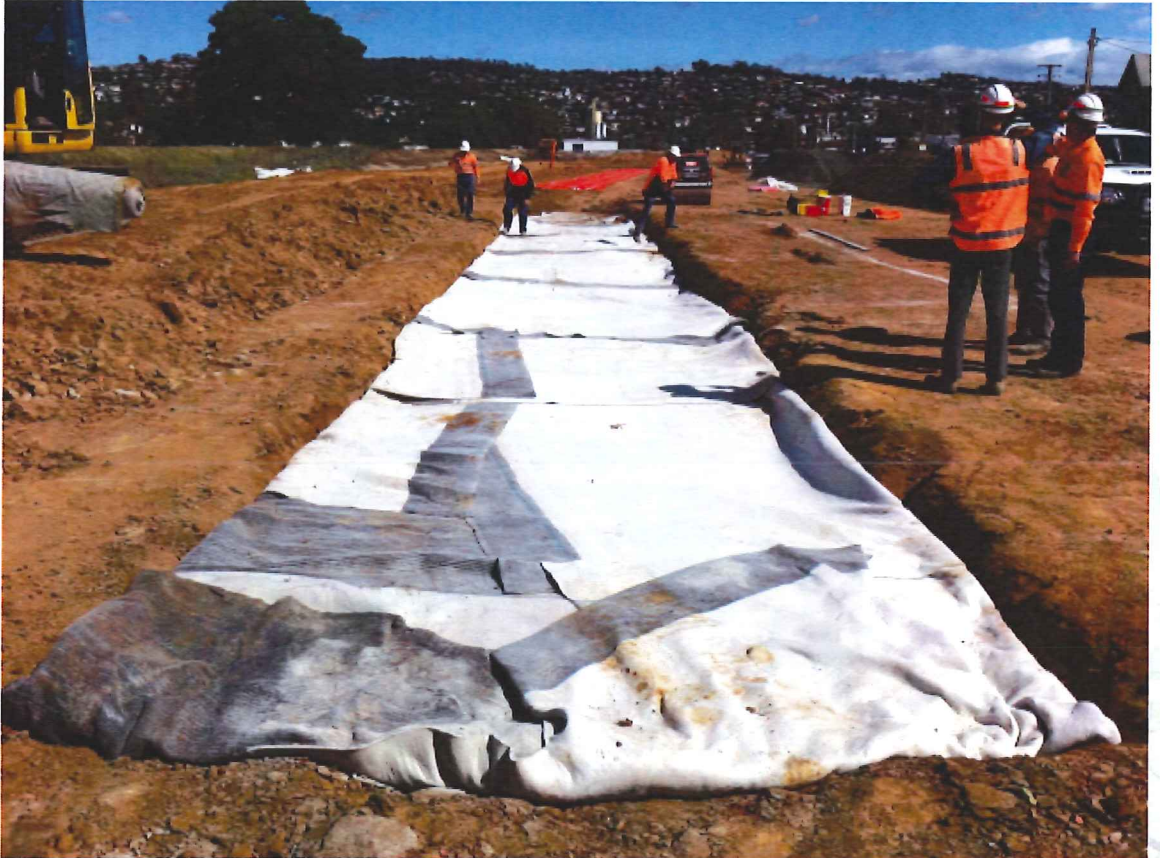
Figure 5: Material wrapped and pinned in geofabric.
