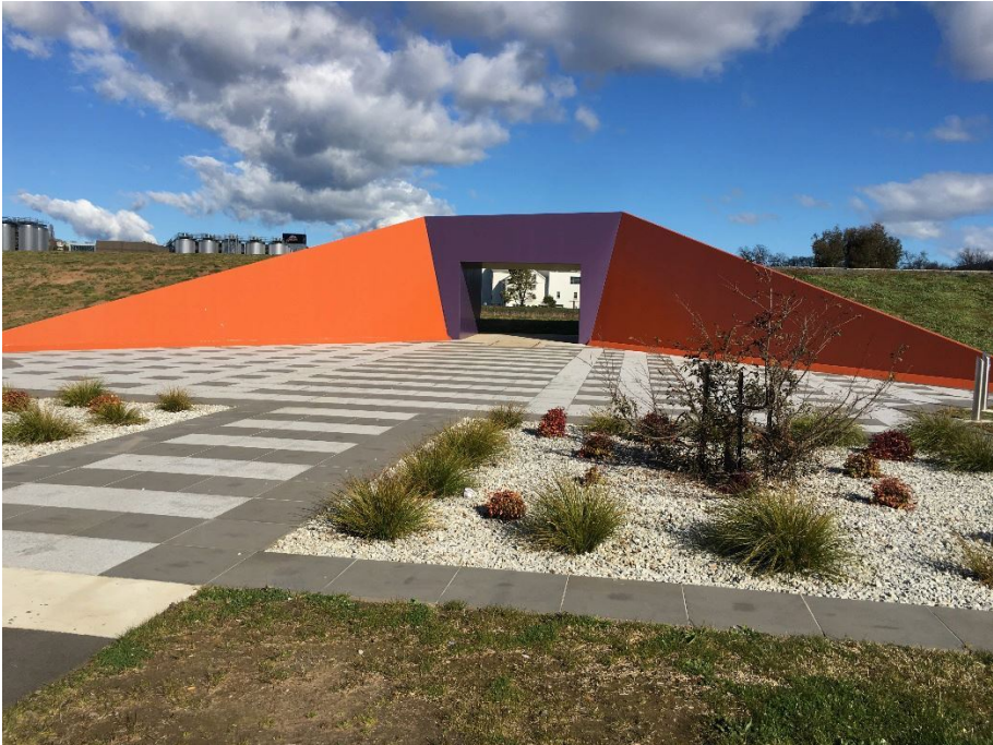
Photo 2 – View of levee underpass (to be retained).
