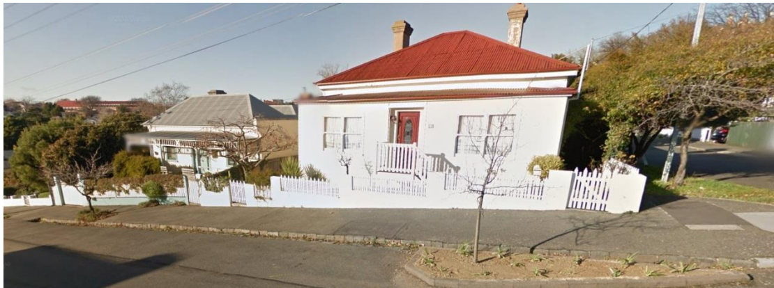
Figure 9: Retaining walls across the frontage in Ann St
