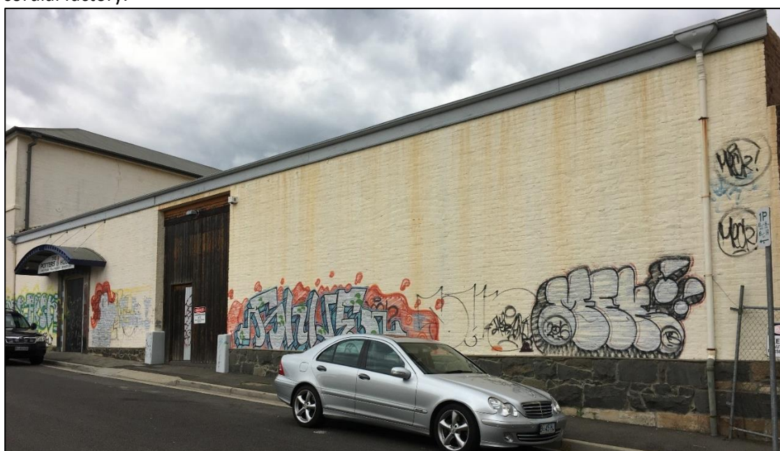
Figure 4 the wall connecting 16 Charles St to the old cordial factory – this will be reduced in height to a minimum of 1500 mm in the left of the photo with steel features to mark the openings
