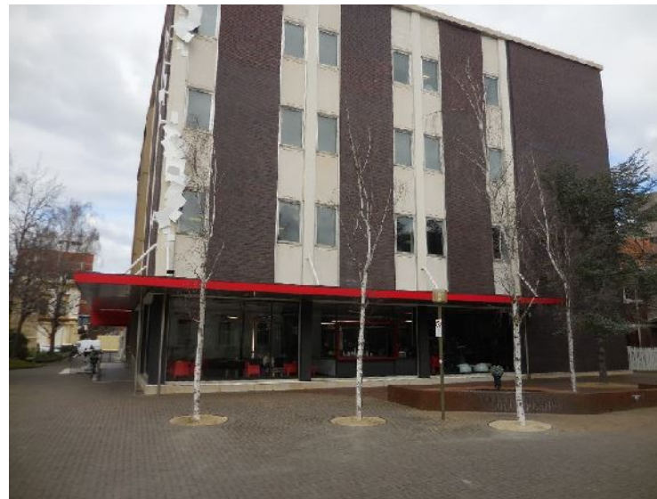
Fig. 9 The poor performing birches and cedar growing in concrete pipes in front of LINC.
