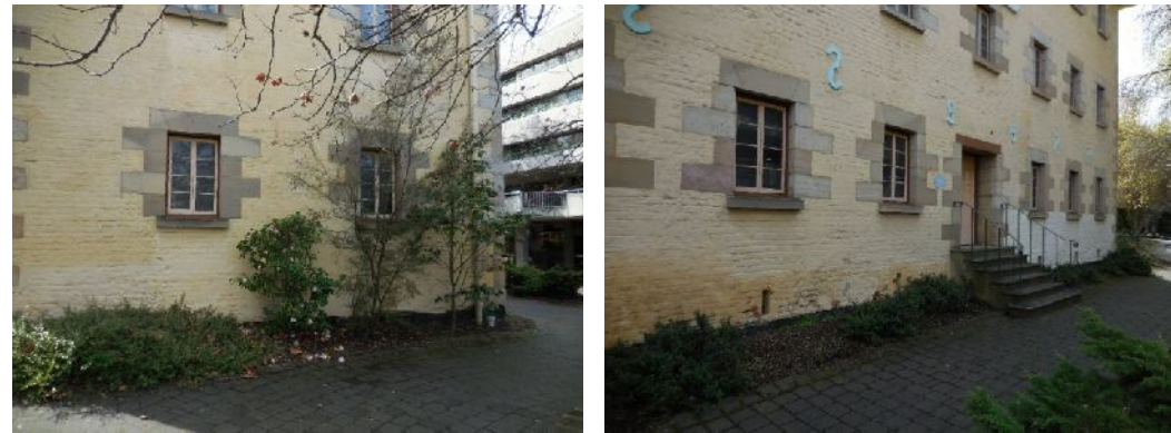
Fig 3. The western and southern side of Macquarie House.
