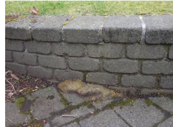
Fig 2. From left: the broad-spreading crown of the plane provides a strong landscape element and welcome shade over the summer; the garden edge and light are being displaced by large roots; a root squeezing below the south-eastern section of the low retaining wall.
