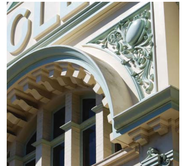
Quadrant Mall Building Façade Detail
