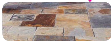
Feature paving at strategic locations
