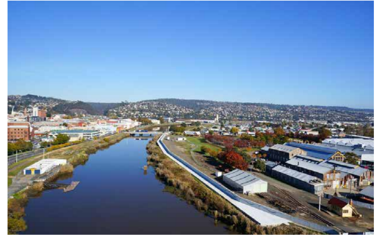
Aerial view of new levee works along the northern edge of the river.
