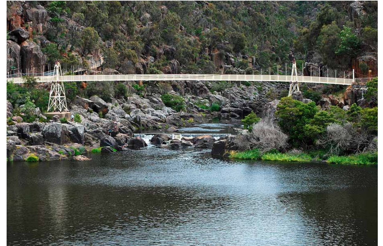
Alexandra Suspension Bridge
