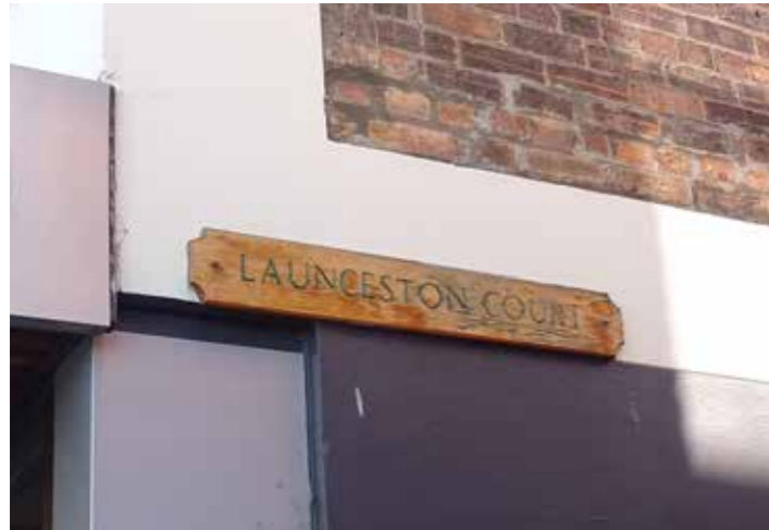
Wooden sign mounted to building. Weathered and cracked wood, alongside minimal contrast between board and letters reduces legibility from distances.
