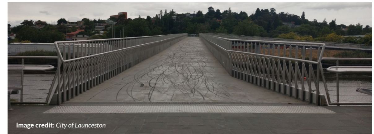
Figure 12. Tyre marks, UTAS pedestrian bridge (Jan 11th 2022)
