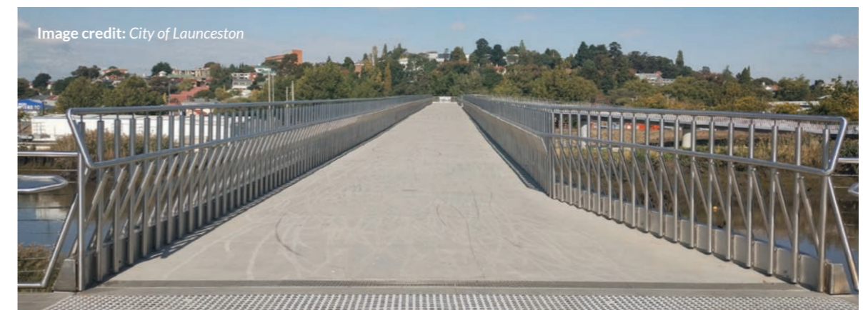
Figure 13. UTAS pedestrian bridge, 8 weeks after cleaning and changes made by operators
