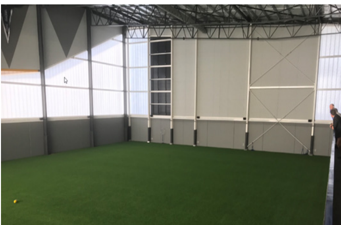
Indoor Training Facility at West Coast Eagles High Performance Centre
