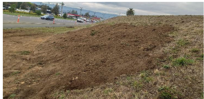
Figure 5. Photos of crack repairs and reinstatement on Kings Wharf Levee, April 2019
