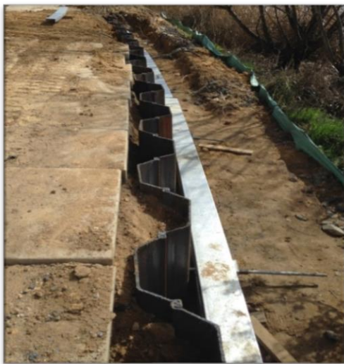
Figure 1. Invermay Levee Stabilisation with steel piling and tie rods, October 2018
