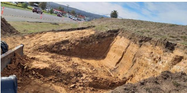
Figure 5. Photos of crack repairs and reinstatement on Kings Wharf Levee, April 2019
