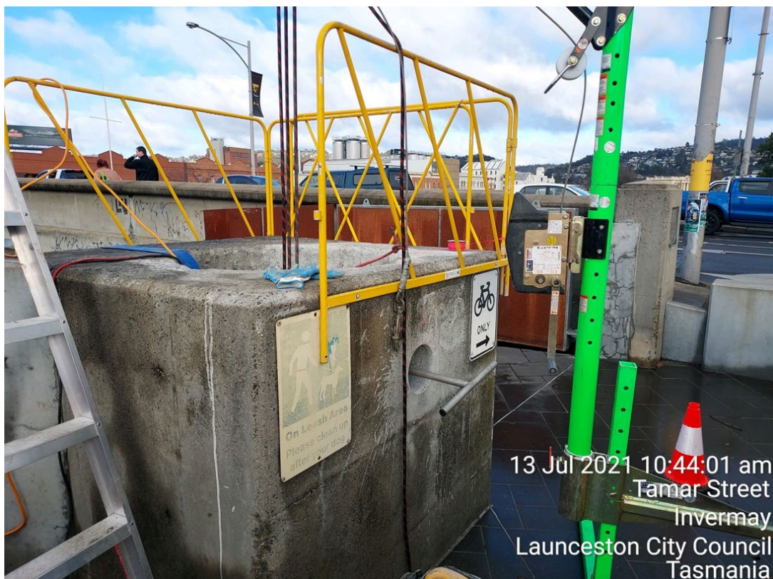
Figure 7 - Invermay Levee - Access Shaft to Renewed Penstock (IP1) - Key (Handle) for Penstock Closure Visible on Side of Shaft
