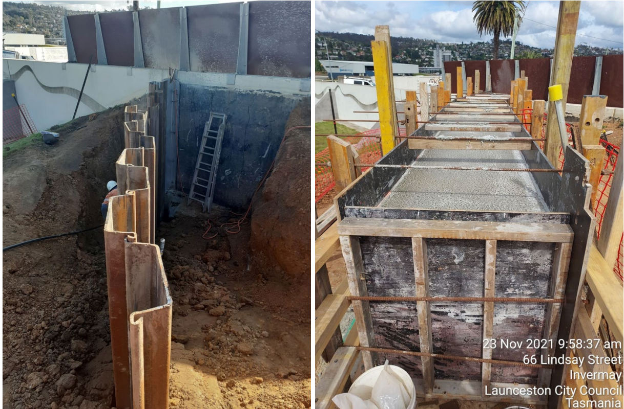
Figure 5 - Installation of the Concreting Capping Beam Over the Steel Sheet Piling - November 2021
