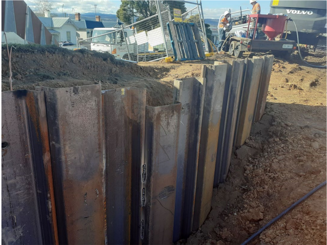
Figure 3 - Sheet Piling Installation (August 2021)
