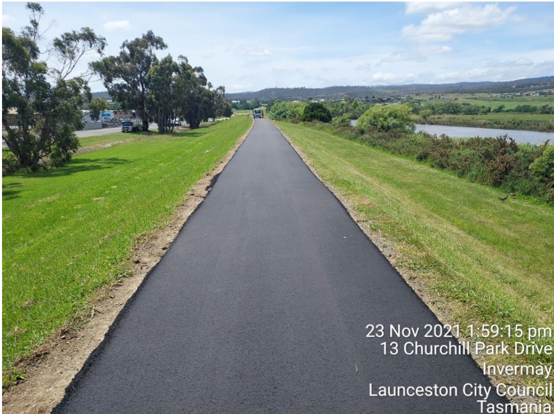
Figure 8 - Newly Sealed Footpath, Invermay Levee (November 2021)
