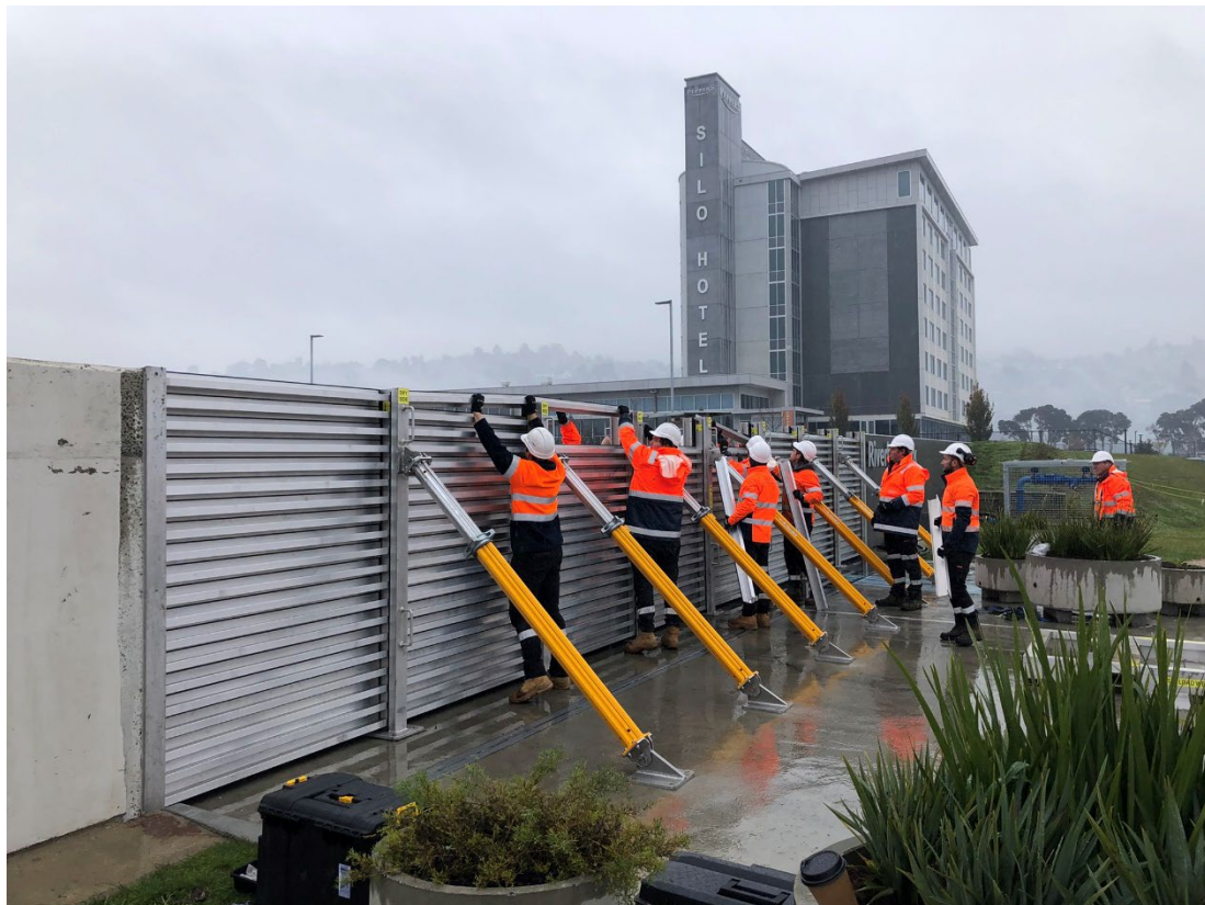
Figure 11 - Floodgate Closure Exercise - June 2022
