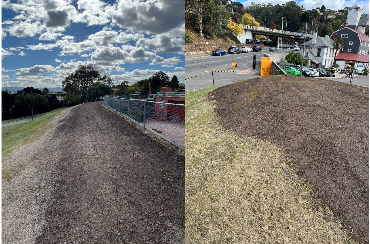
Figure 2 - Paterson Levee Top Soil and Reseeding - April 2022
