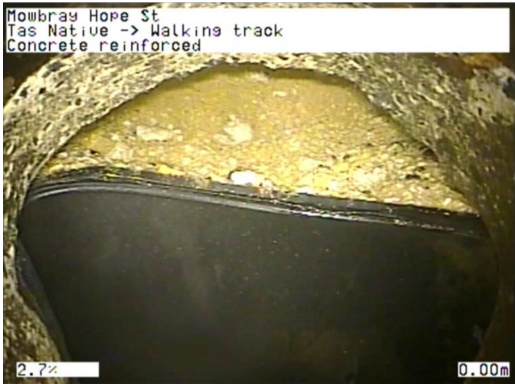
Figure 9 - Collapsed Pipeline at MP1 Chamber, Internal CCTV Footage showing pipeline (black) and levee clay from inside access shaft.
