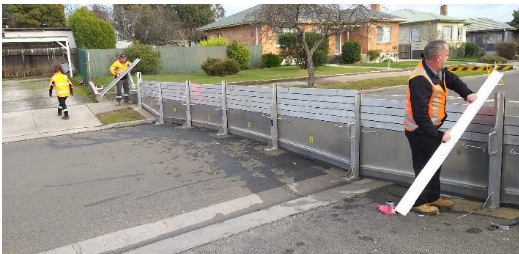
Figure 2. Newstead Levee floodgate test installation, July 2019
