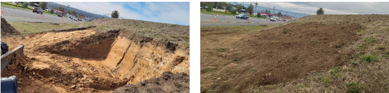
Figure 5. Photos of crack repairs and reinstatement on Kings Wharf Levee, April 2019
