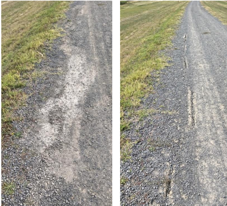
Figure 4. Photos of crack repairs with bentonite slurry Invermay Levee, March 2019
