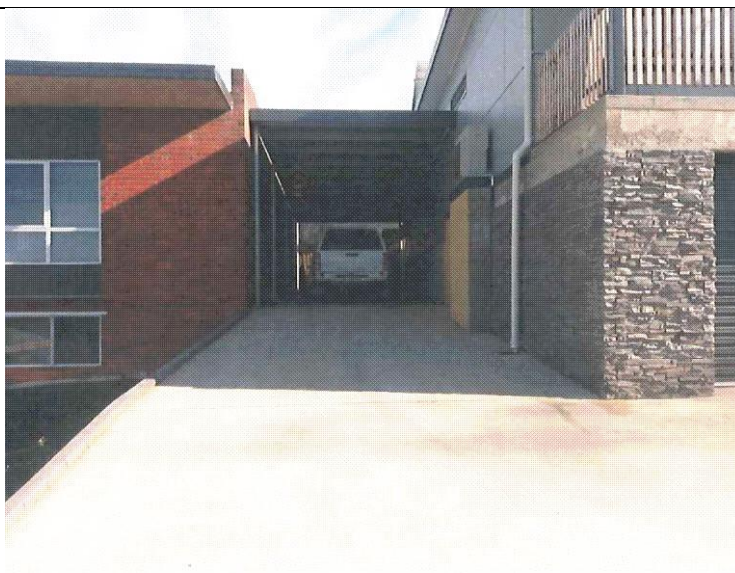
Figure 2 - Constructed retaining wall
