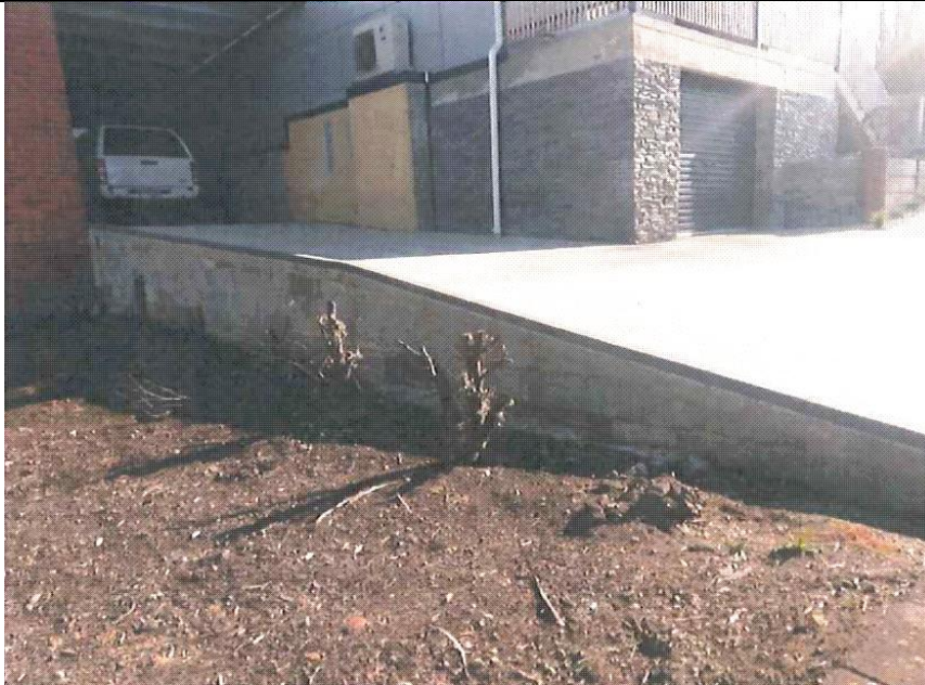
Figure 3 - Existing Retaining Wall
