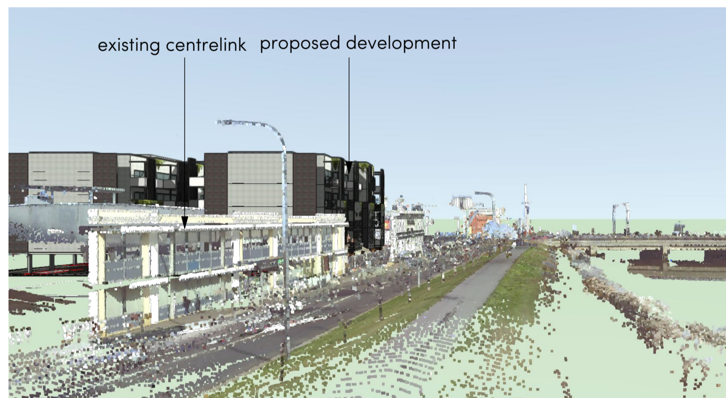
view from levee bank towards Tamar St
