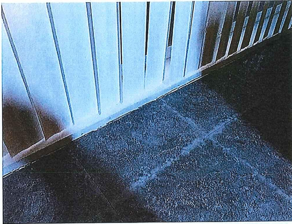
Photo 23 - Photo in kitchen/dining area - slight movement noted between flooring and window
