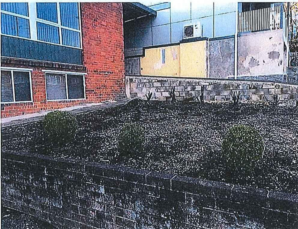
Photo 2 - Photo looking north from driveway. Note concrete block driveway retaining wall for 27 Benvenue Road.
