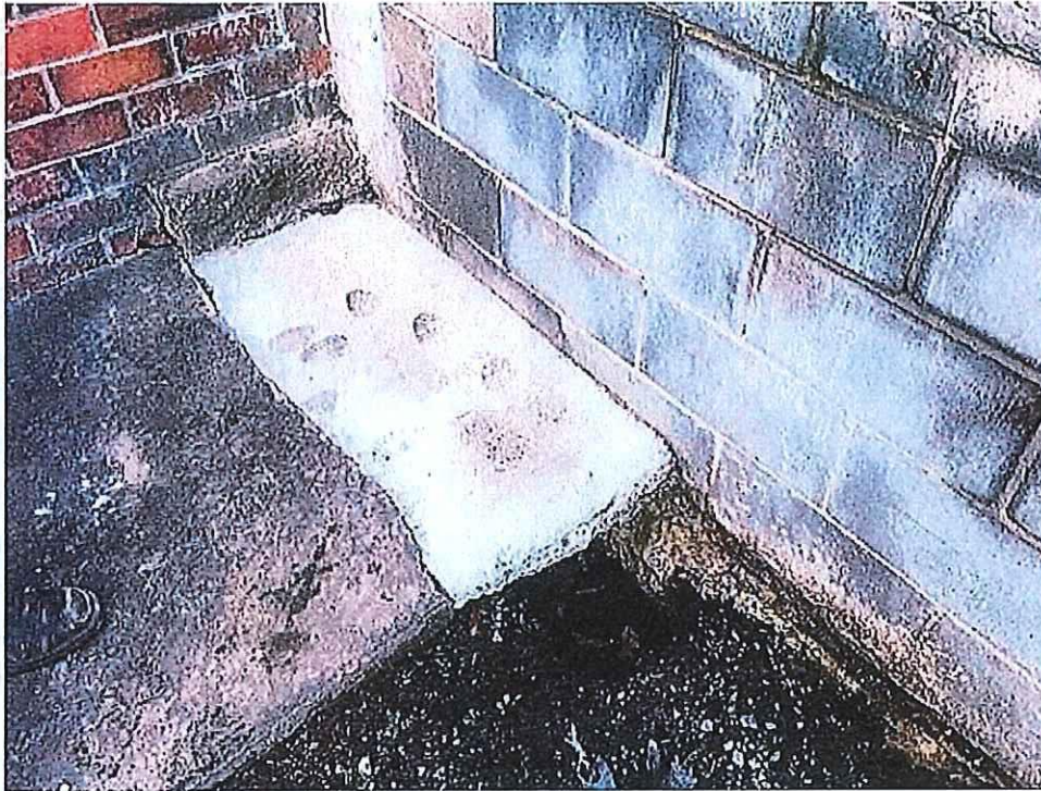
Photo 5 - Photo showing intersection of boundary retaining wall and brick wall. Note concrete works performed as part of construction works for 27 Benvenue Road.
