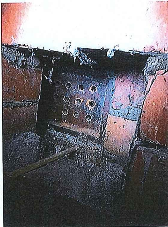
Photo 20 - Sub-floor ventilation on north east boundary wall which has been blocked by construction of neighbouring driveway.
