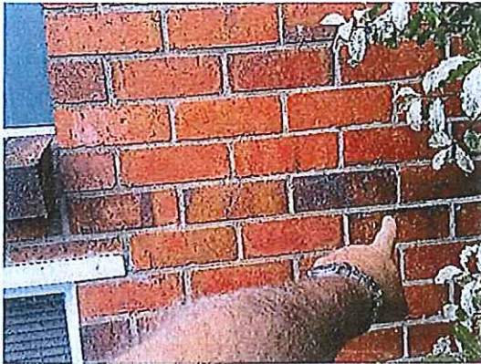
Photo 7 – horizontal cracking extends back to near the window on this front elevation.
