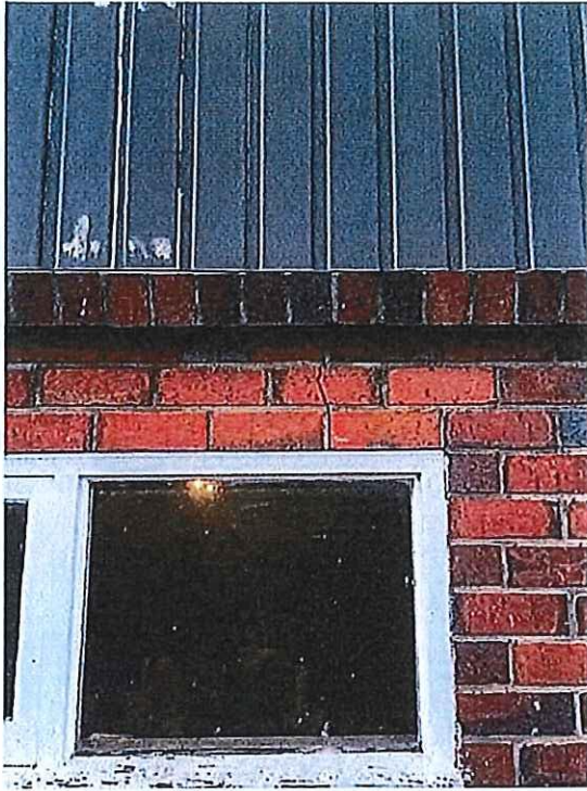
Photo 14 - General view of south west face at location of crack shown in Photo 13 and movement to timber cladding.
