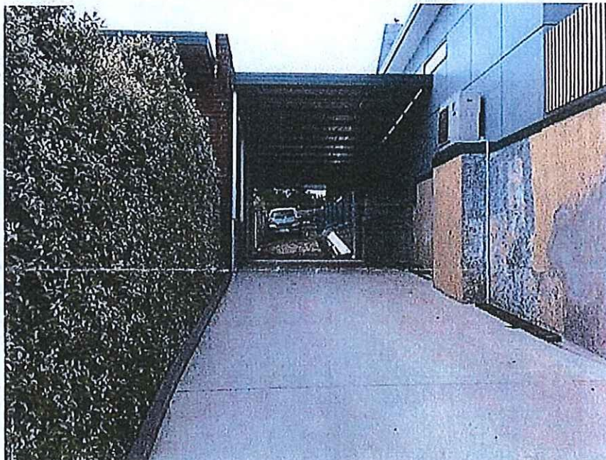
Photo #1 - Carport and concrete driveway at 27 Benvenue Road.
