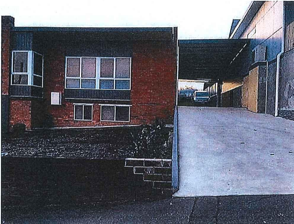
Photo 1 - Photo looking north west along the property boundary. on the left, 27 Benvenue Road on the right - note new concrete driveway and carport.
