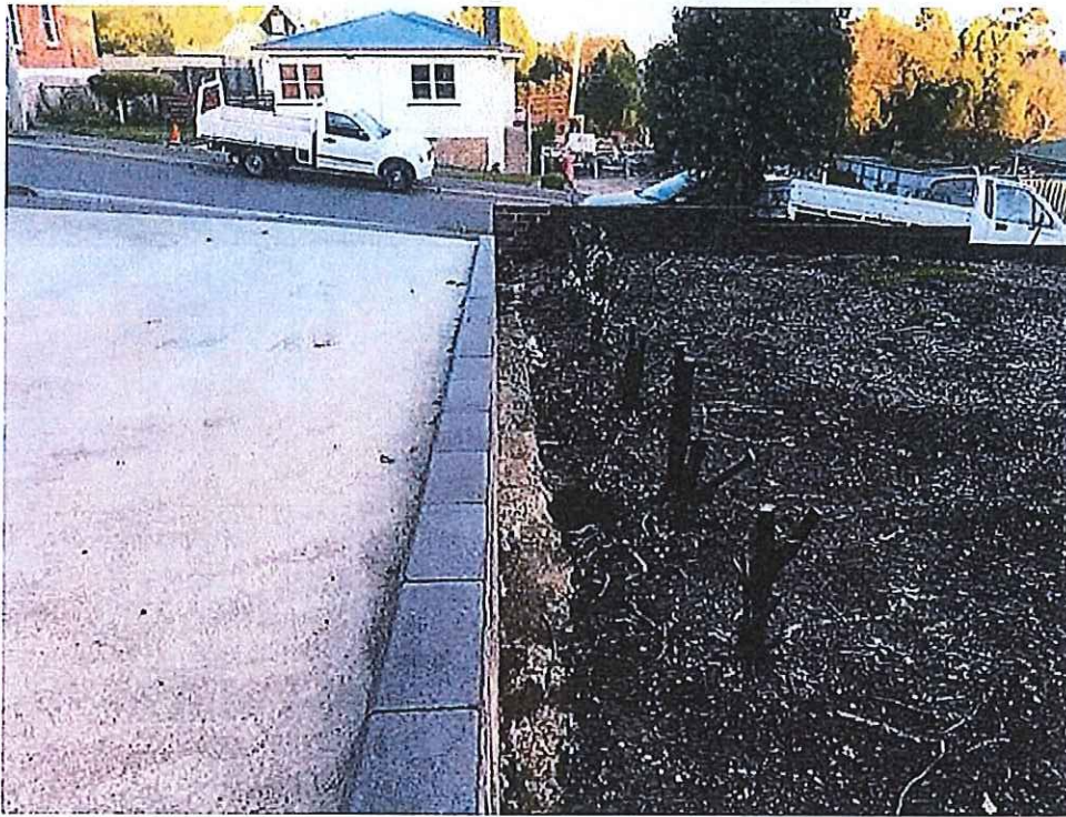
Photo 9 - Photo looking south east along property boundary retaining wall. Note paved kerb against boundary wall.
