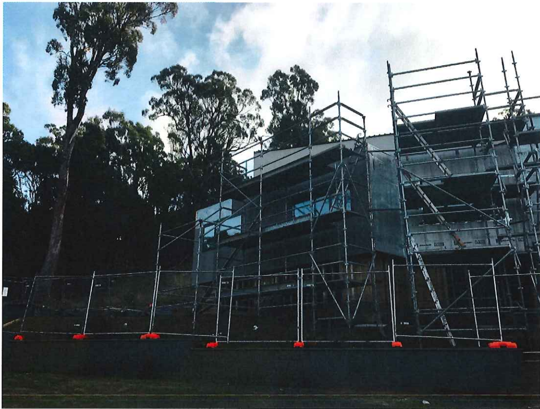
FIG.11 PHOTOS OF NEIGHBOURING DWELLING FROM BACKYARD
