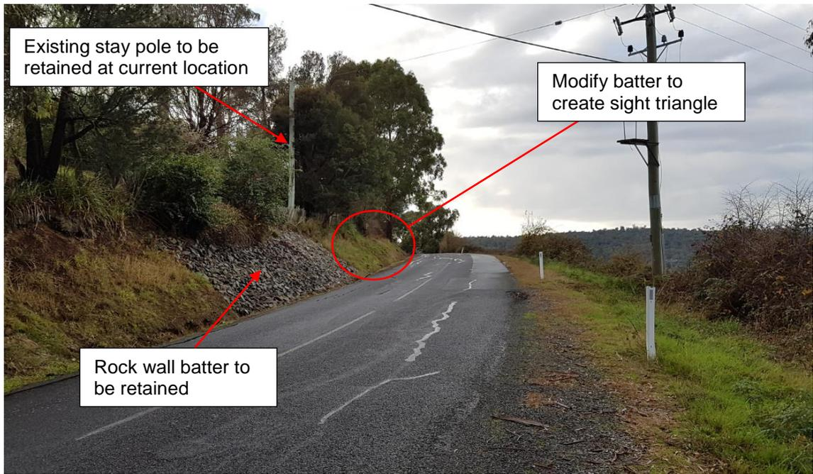
**Figure 7 Recommended Batter Works**
