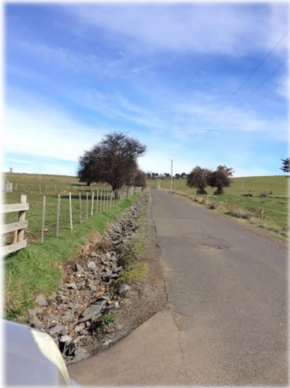
Figure 3 – Boomer Road at existing residential access, looking left towards Tasman Highway
