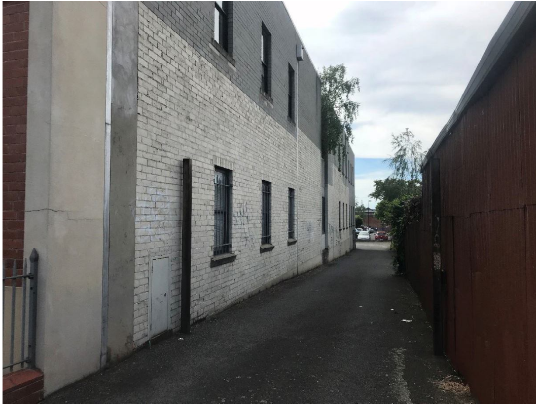
Photo 7: Eastern elevation of 10-14 Cameron Street
