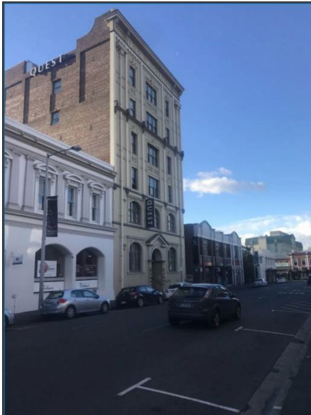
Photo 5: Scale of Question building in comparison to adjacent properties
