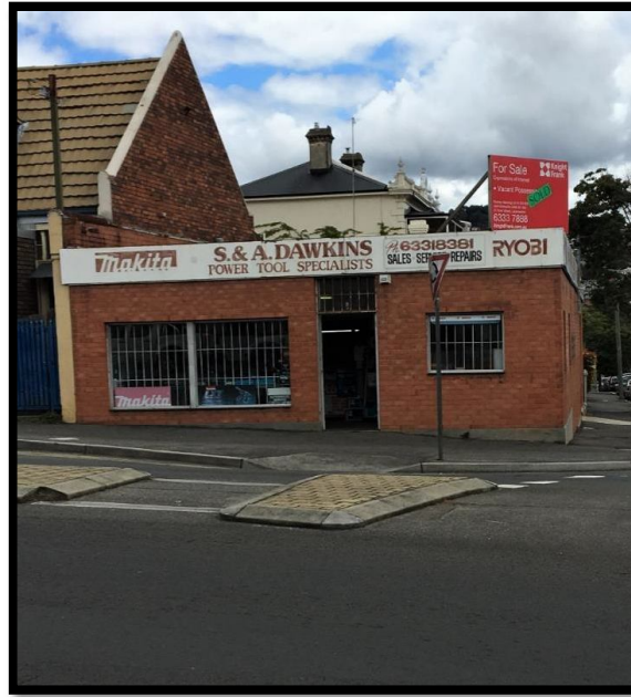
Figure 3: Existing Charles Street Elevation
