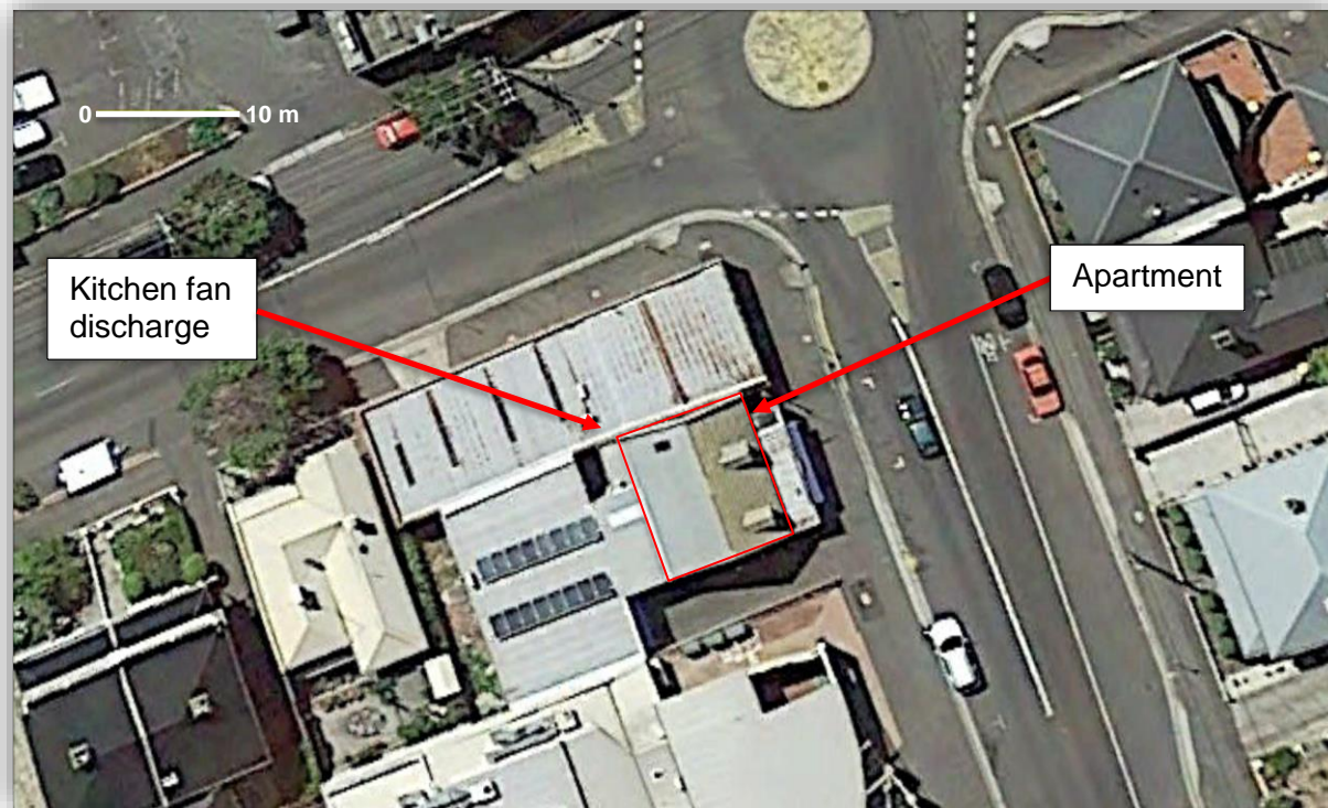
Figure 6 – Aerial view of apartment at 256 Charles St.
