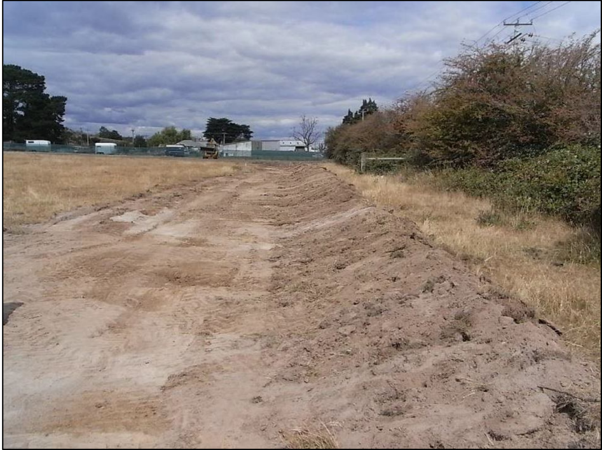
Figure 12 – Constructed bund completed on 20 th February 2017
