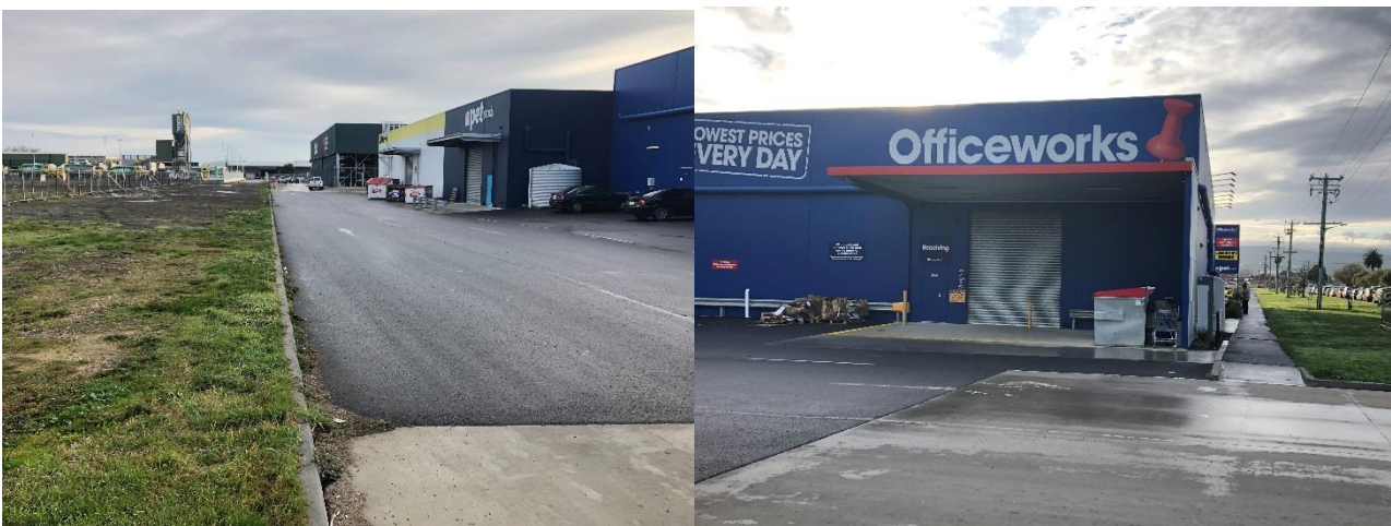
Figure 2 - Officeworks and other similar developments adjacent to the site
