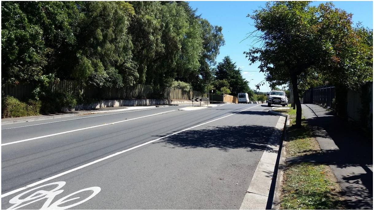
Figure 3 Elphin Road looking north
