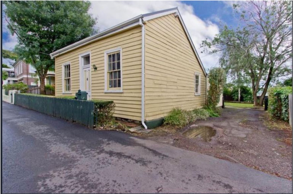
Existing cottage to Middle Street - view to access drive & mature tree (to remain)
