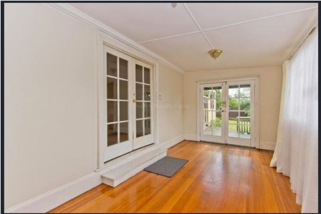
Access to new extension via existing door to right side of fireplace - remove existing firebox & flue. Block off door into existing rear skillion and install new double doors onto new deck - refer plan
