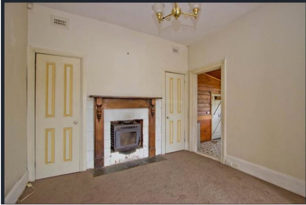
Access to new extension via existing door to right side of fireplace - remove existing firebox & flue. Block off door into existing rear skillion and install new double doors onto new deck - refer plan
