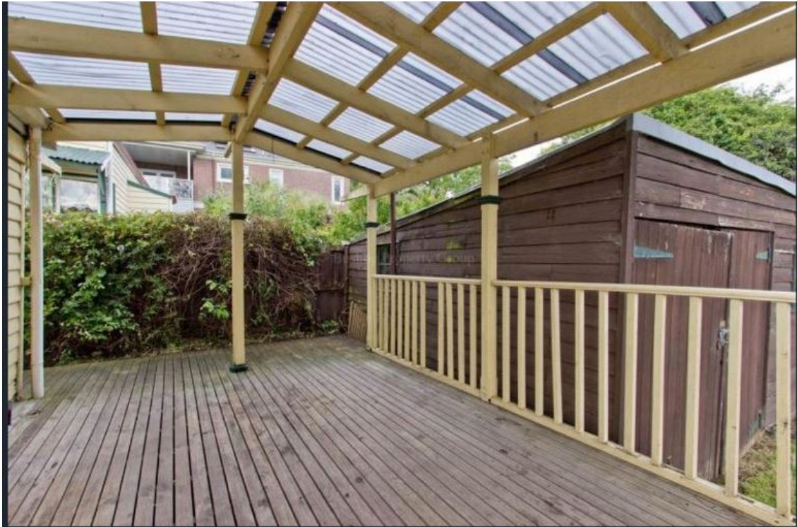
Existing covered deck & outbuilding to be demolished View from north eastern corner of site - grey pitched roof to be retained
