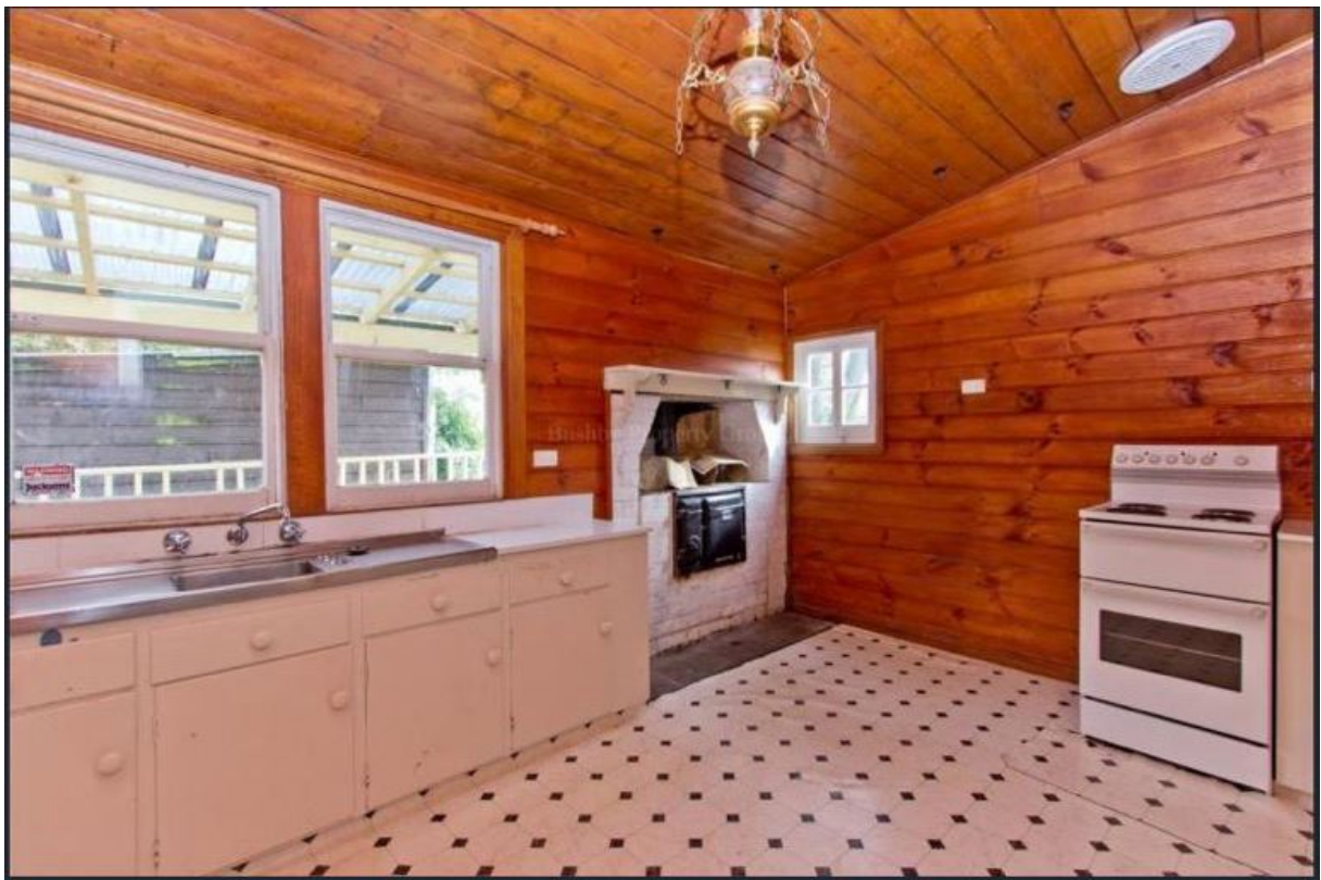
Rear skillion - kitchen/laundry room - to be demolished
