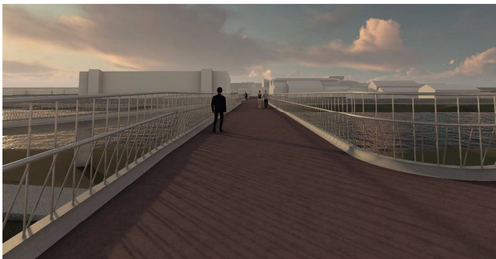
Figure 1 Artists impression of the deck of the bridge showing hand rail and bicycle guard rail
