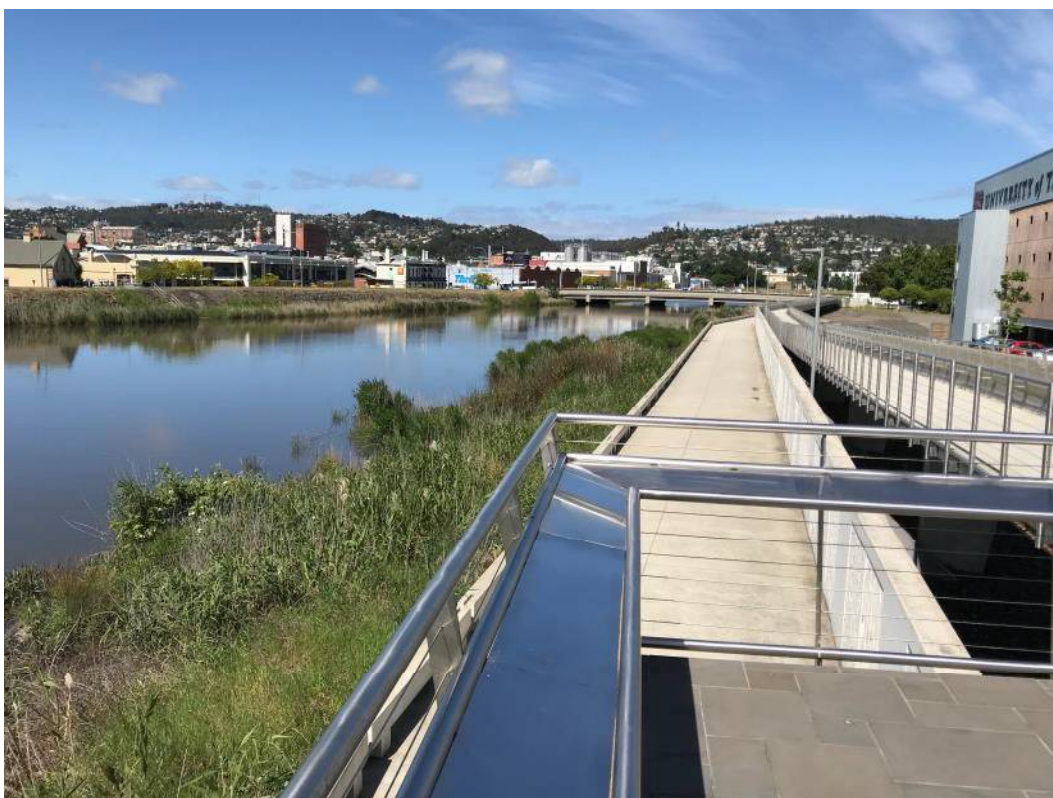
Plate 4 View west along the north bank of the North Esk River from the existing pedestrian access over the foreshore pedestrian-cycleway fronting the UTAS Campus
