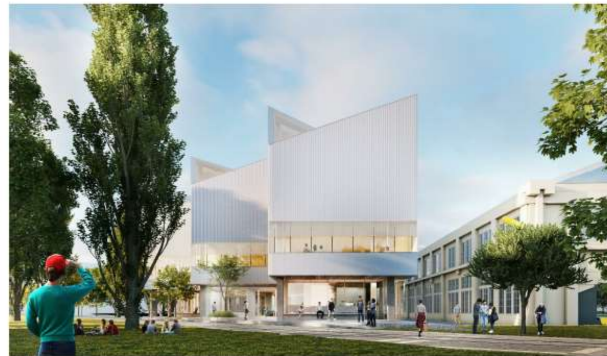
VIEW FROM SOUTH WEST
