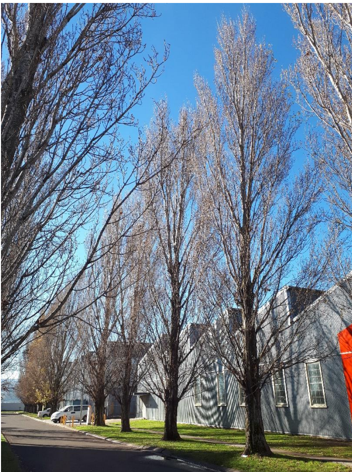
Trees 5 - 8 (foreground to background). Note the distance to, and height above the building. Due to the design of the gutter system, there are no practical solutions to avoid their constant blocking with tree debris in Autumn.
