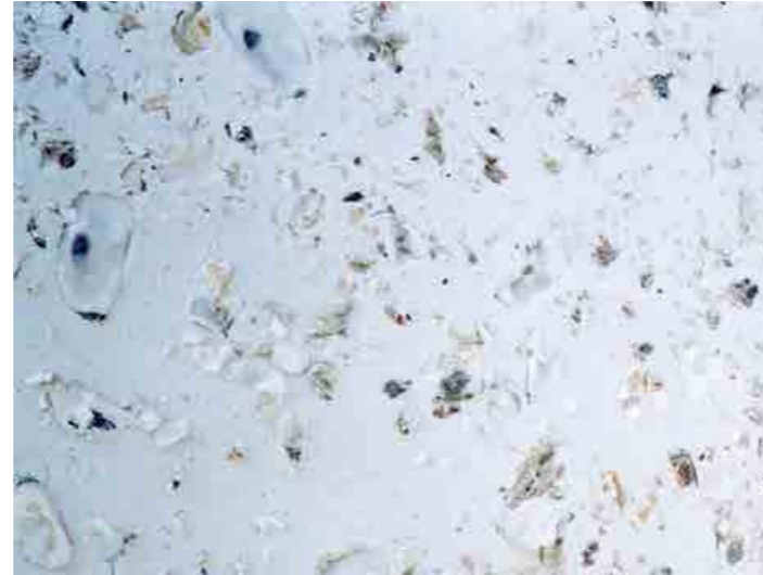
Insitu concrete with sea shell aggregate
