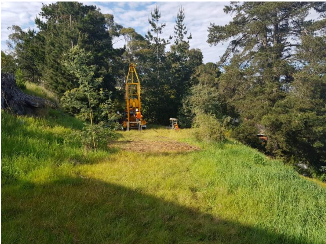
PLATE 2 - THE CUT TO FILL BENCH LOOKING TO THE SOUTH
