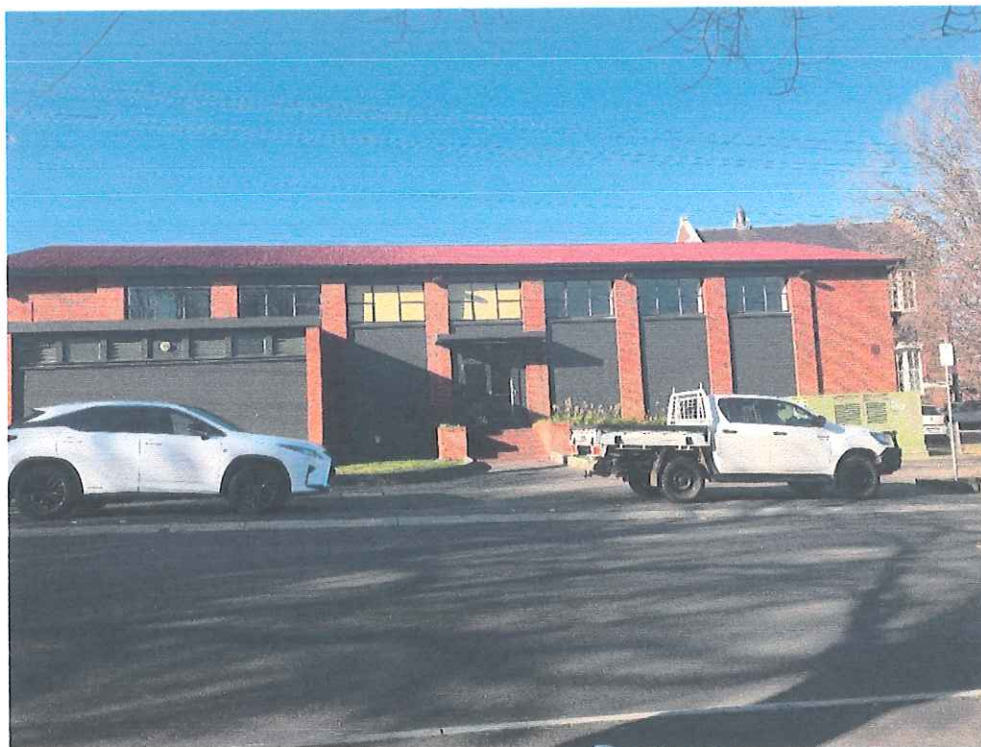
Figure 3 Subject site from Canning St
