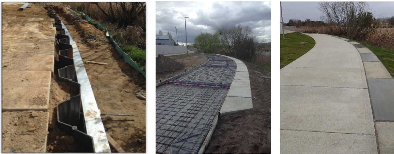
Figure 1. Invermay Levee Stabilisation with steel piling and tie rods, October 2018
