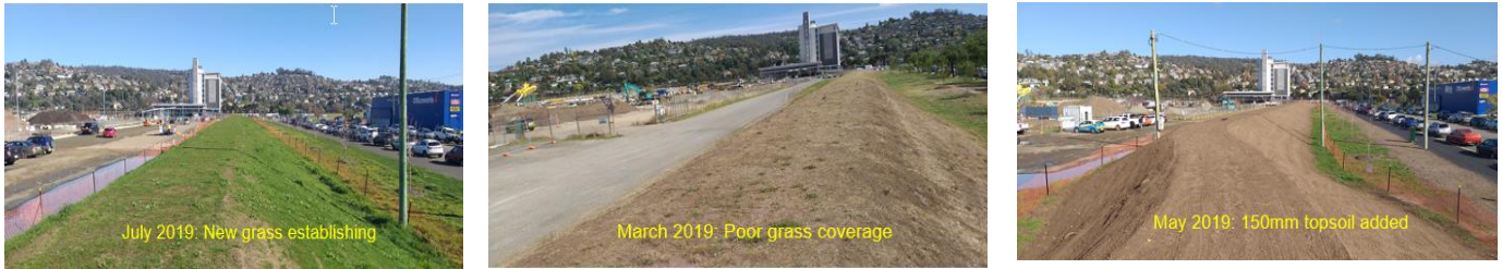
Figure 6. Photos of grass repairs on Kings Wharf Levee, March to July 2019
