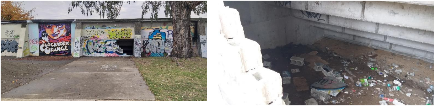
Figure 8. Photos of vandalised besser block wall panel, May 2019
