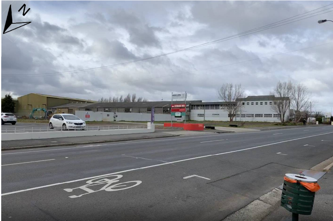
Figure 19: Looking southeast towards the Charity Shop, T&G Flooring, ACL Bearings and the former James Nelson building.
