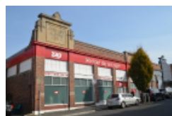
Intact façade on adjoining title - No.2 Kingsway
