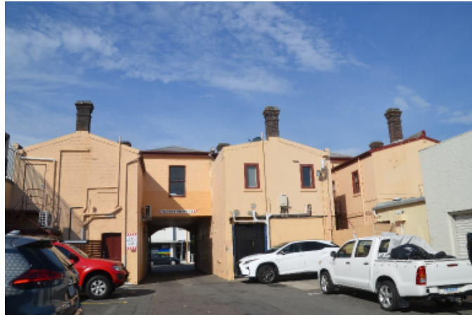
Rear of the Building (192 and carriageway at left)
