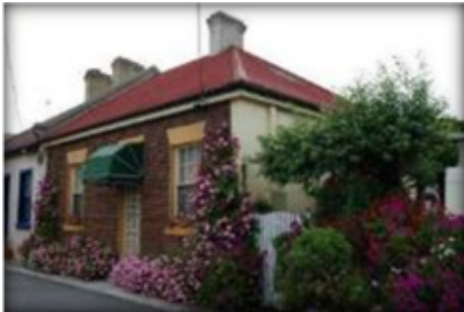
Kilby Lane streetscape Launceston City Council
