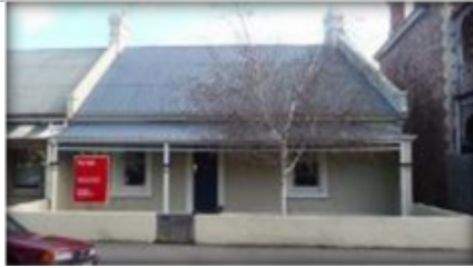
Martin Boland's residence, 28 Cimitere Street
