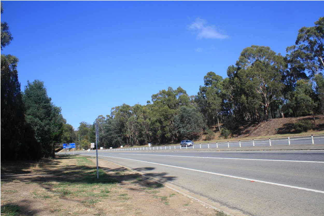
Figure 9: Mature trees providing vegetative screening.
