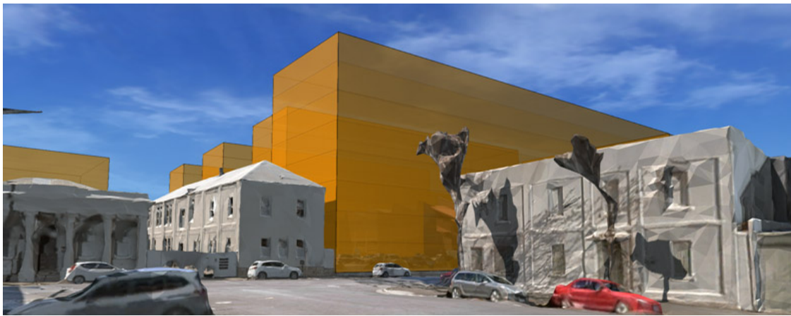
Figure 64: SITE B1 - Option 2 - View looking south along Shields Street.
