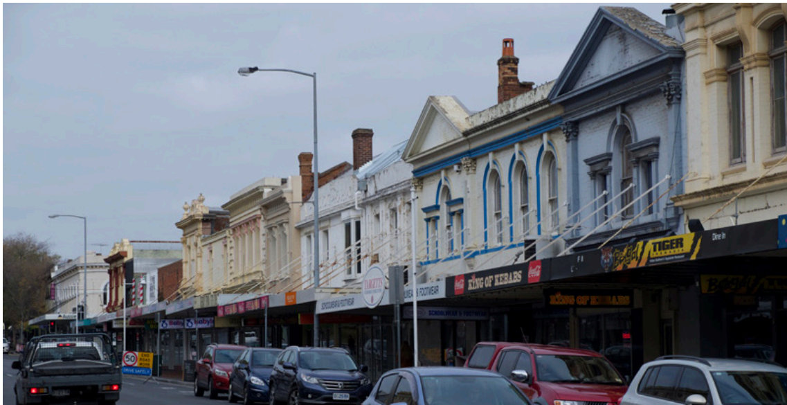
Figure 16: Another streetscape of very consistent forms with newer forms having a lower scale than the typical adjacent buildings. In this location, street front building heights are around 8-9 metres.
