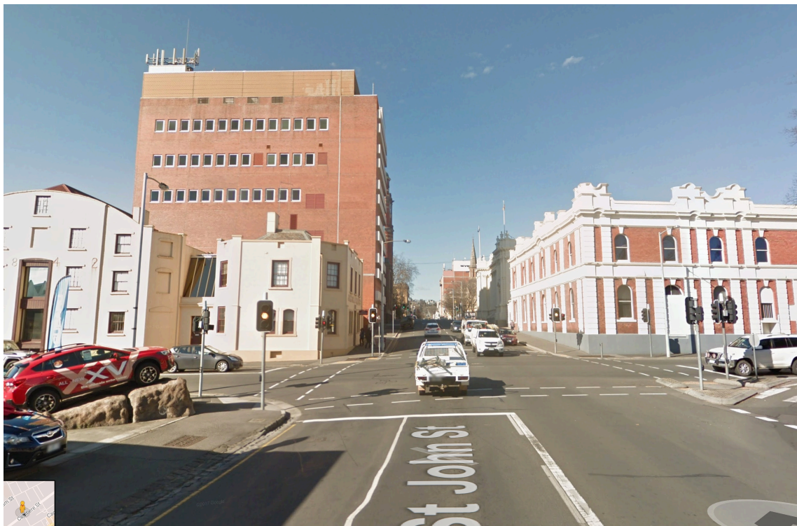
Figure 6: Telstra Building in St John Street. Source: Google Streetview.
