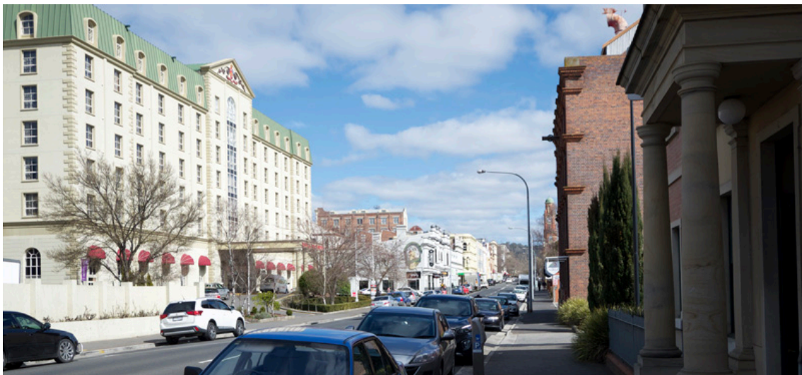
Figure 12: The Grand Chancellor hotel in the context of adjacent development.
