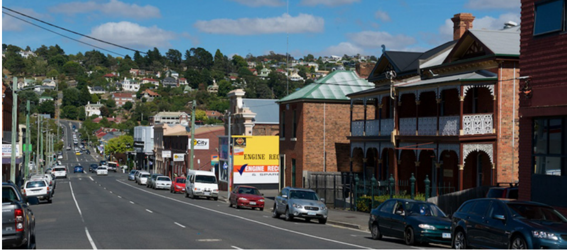
Figure 7: A view west in the southern part of the city along York Street where there is a very consistent two storey scale of older and more recent buildings.
