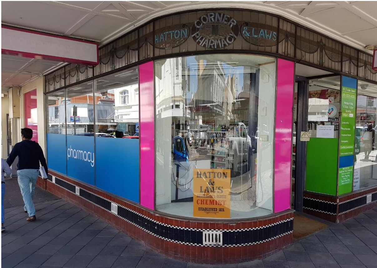
Figure 2: Existing Ground Floor Facade
