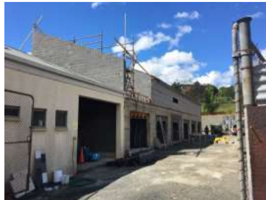
Figure 3: Stage 1 under construction Southern Elevation
