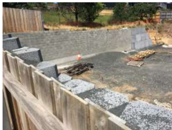
Figure 8: Picture of Retaining Walls
