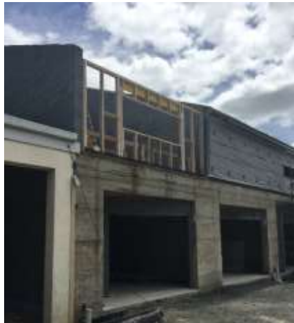
Figure 4: Stage 1 under construction Southern Elevation framing detail
