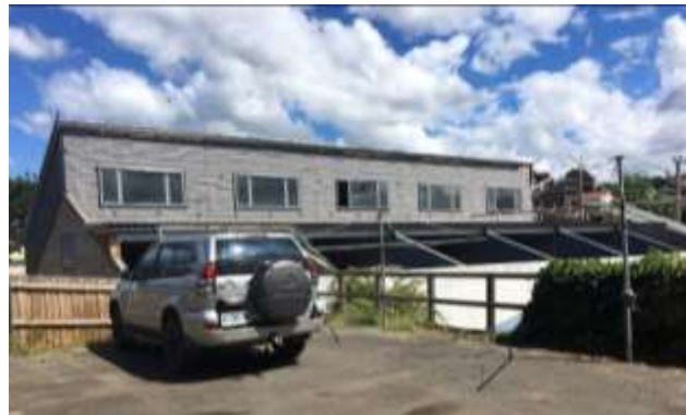
Figure 2: Stage 1 under construction Northern Elevation
