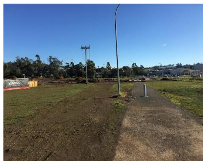
Overview of easement – view south to north
