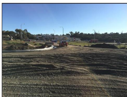
Overview of land – view south to north
