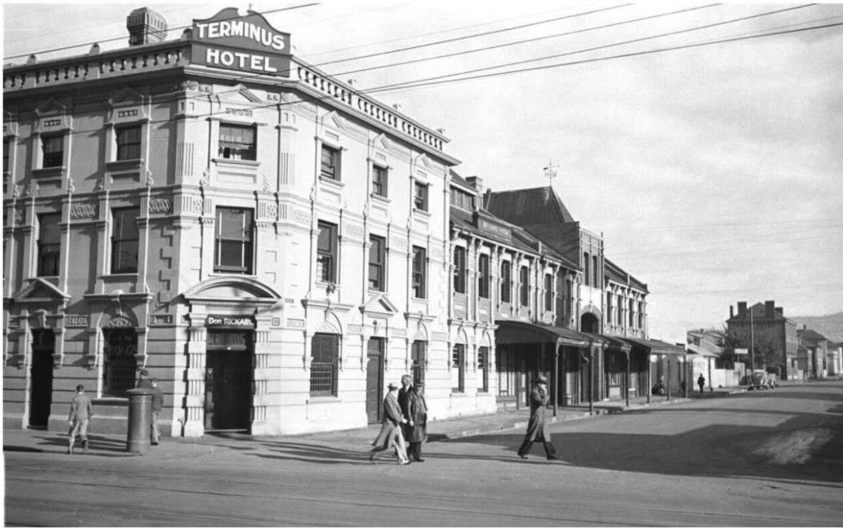
Figure 3.29 – The Terminus Hotel and William Street shops c1950. QVMAG 2006.P.0063
