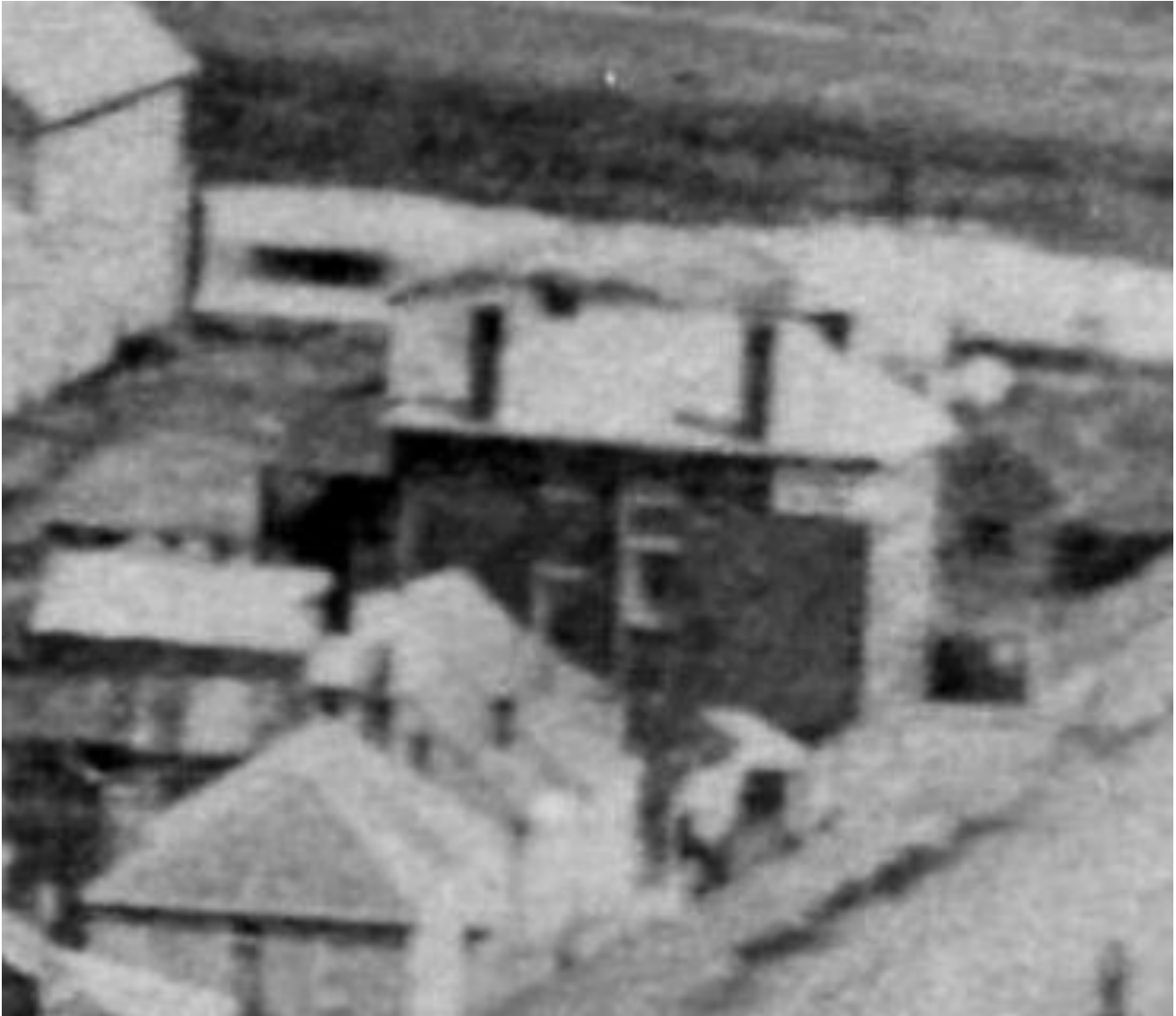
Figure 3.8 – Except from a panoramic photograph of Launceston c1870 showing the Tamar Street frontage and side wall of the Terminus (former Dorset) Hotel. QVMAG.
