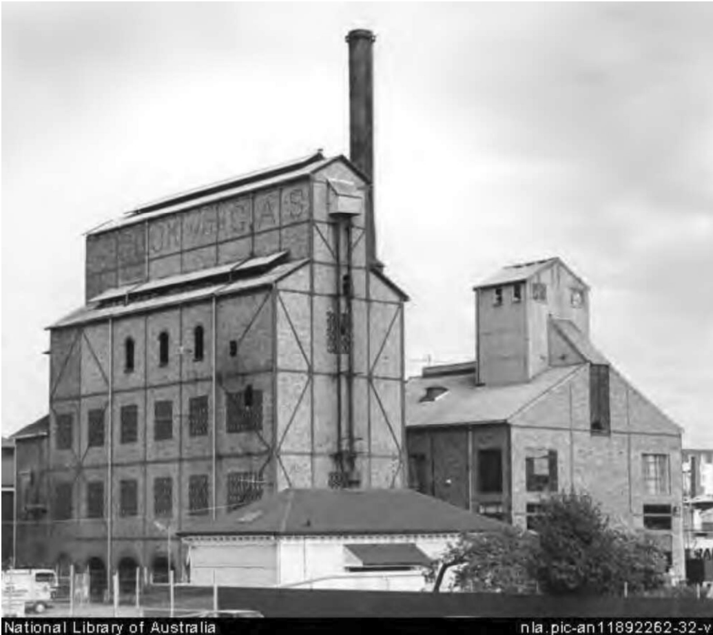
National Library of Australia nla.pic-an11892262-32-v Figure 6 Launceston Gasworks [picture] by Mike Key 1995: https://trove.nla.gov.au/version/27139386
