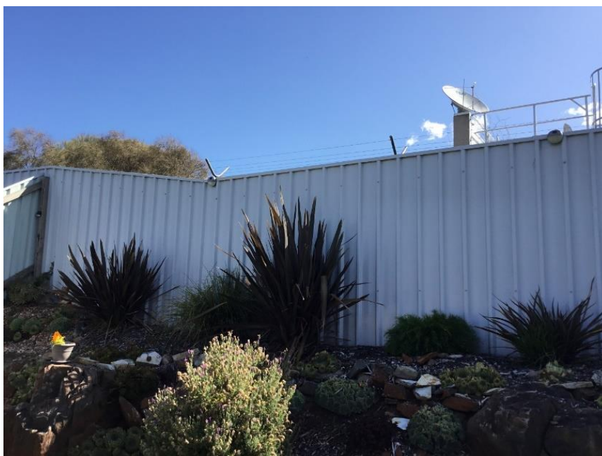
Figure 8 - View of the Site from Rear Garden of Adjoining Lot
