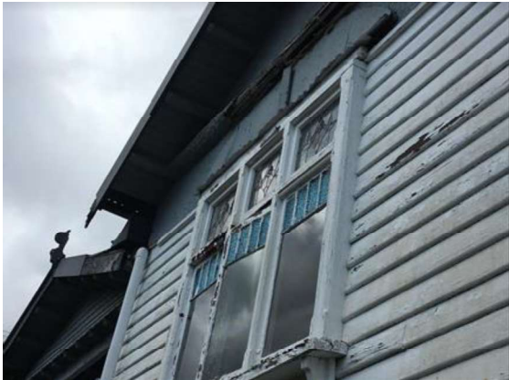
Figure 7: North facing window, the original opening has been patched above the window. Note the failing stucco.
