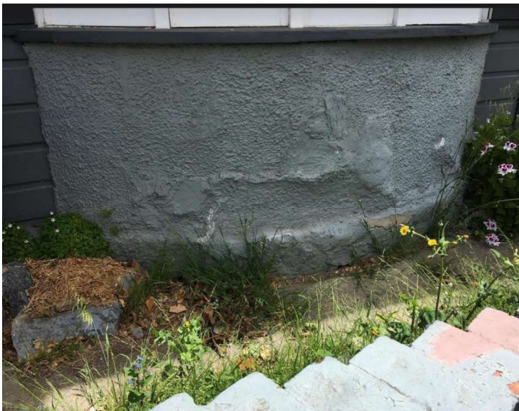
Figure 6: Evidence of subsidence.
