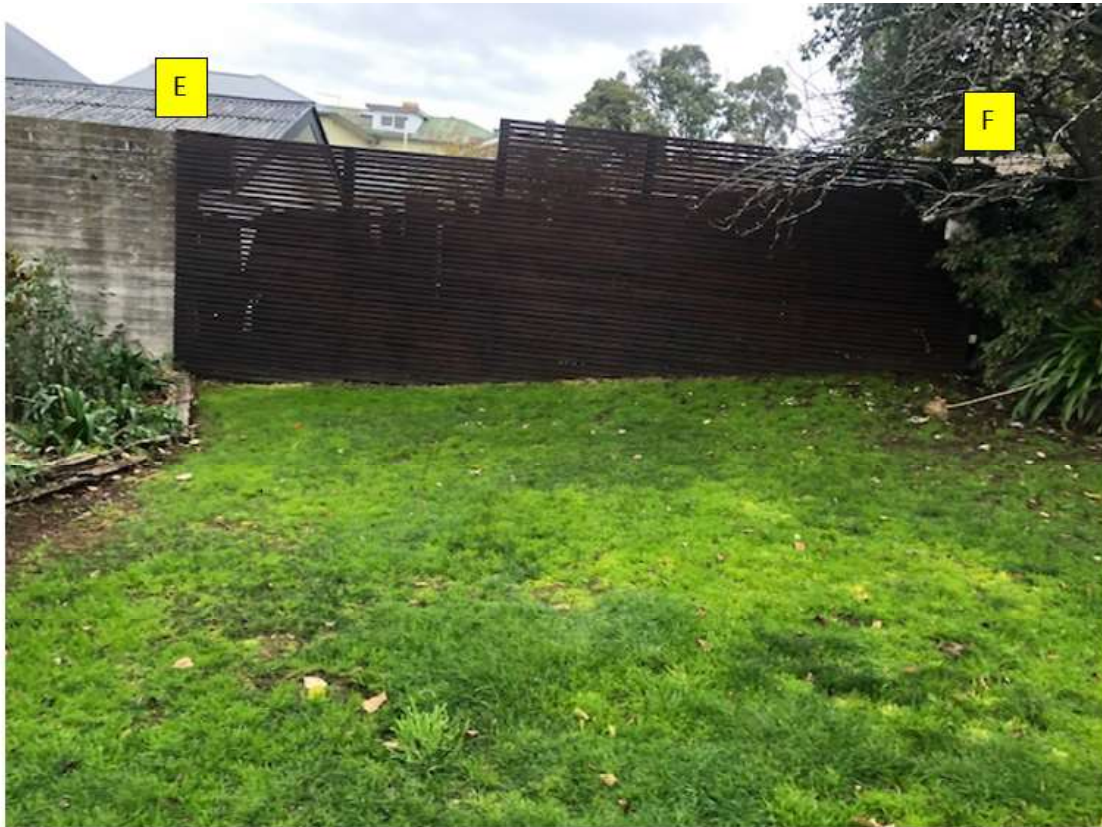
Figure 7 Section E-F Screen fence Jodi erected from concrete wall in front of existing old boundary fence. You can see the old fence behind it.
