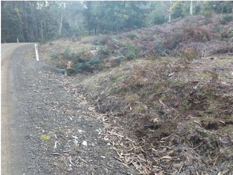
photo 6 Table drain and piped crossover towards the western end of lot
