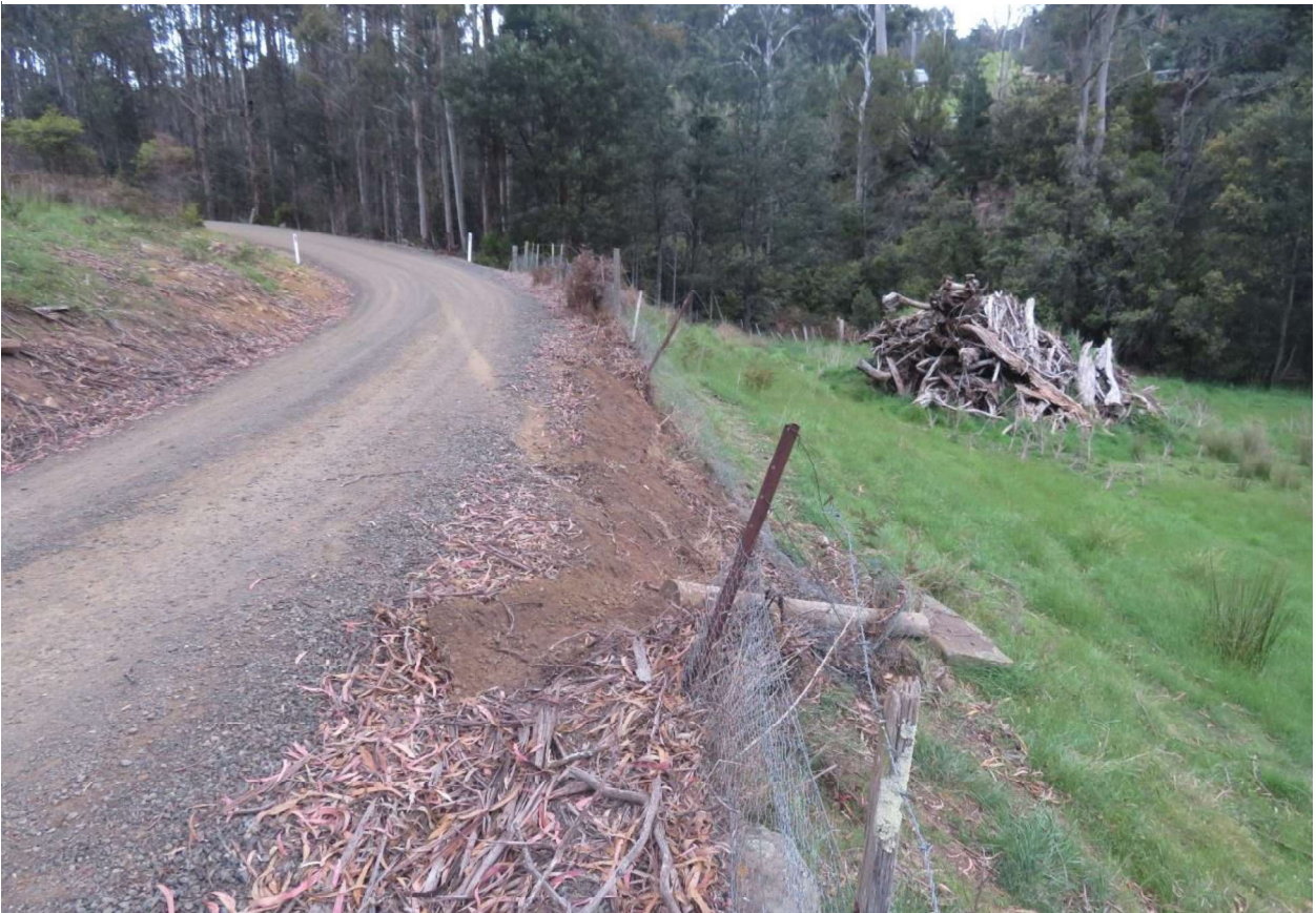
Figure 4. Photo taken after vehicle accident on blind corner please see tyre marks in gravel indicating slide impact.
