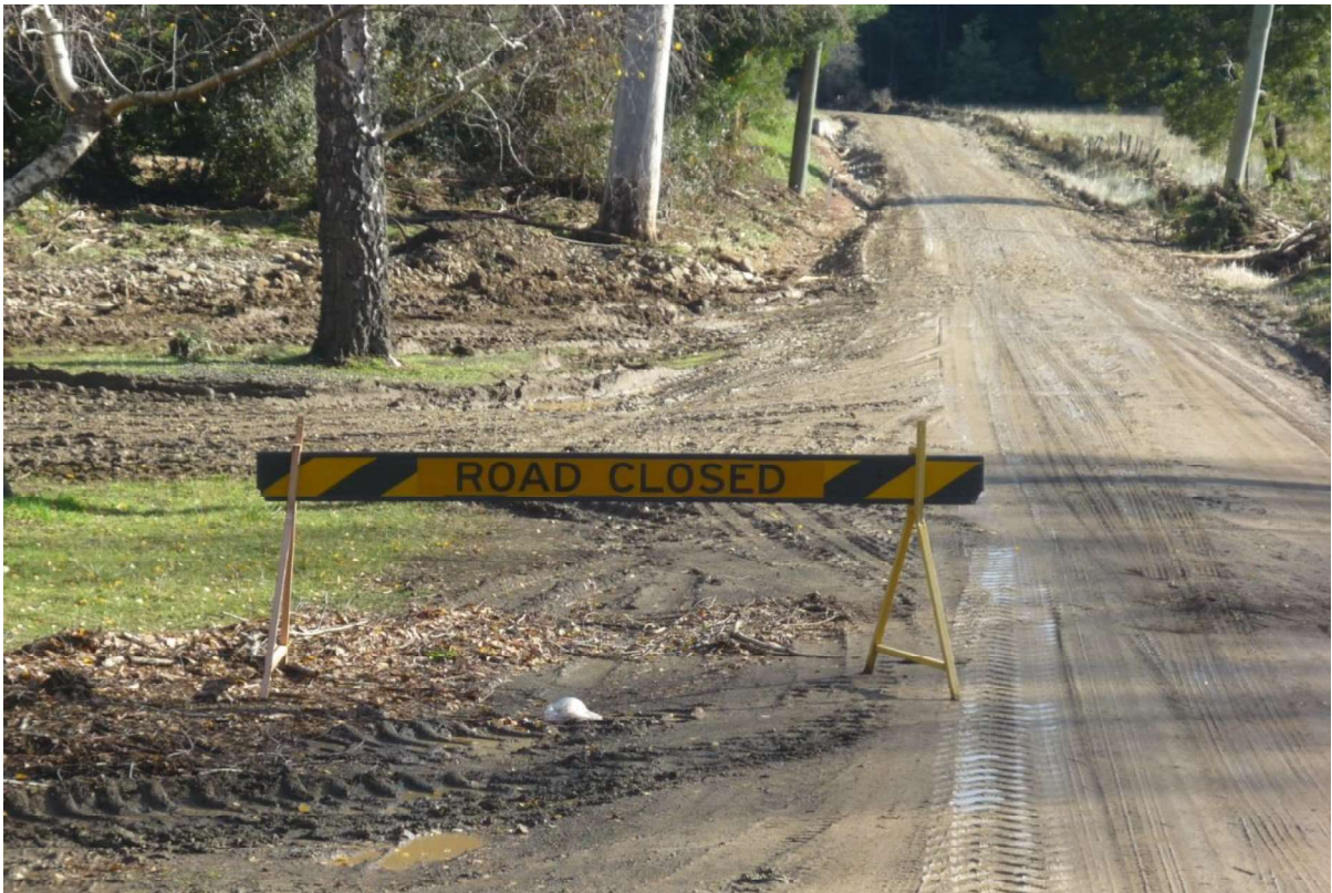
Figure 6. Road closed due to flooding
