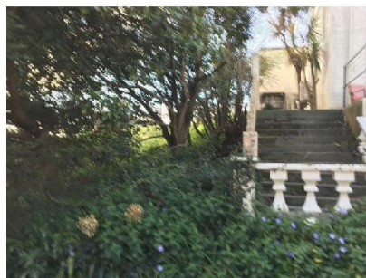
Overview of encroachment
